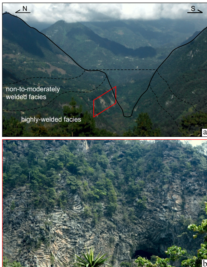
Figure 7: a) North view of the Las Minas valley showing the eroded space and the approximate position of the XI in the different welding facies that changes from highly-welded in the base to non-to-moderately welded through the top.
